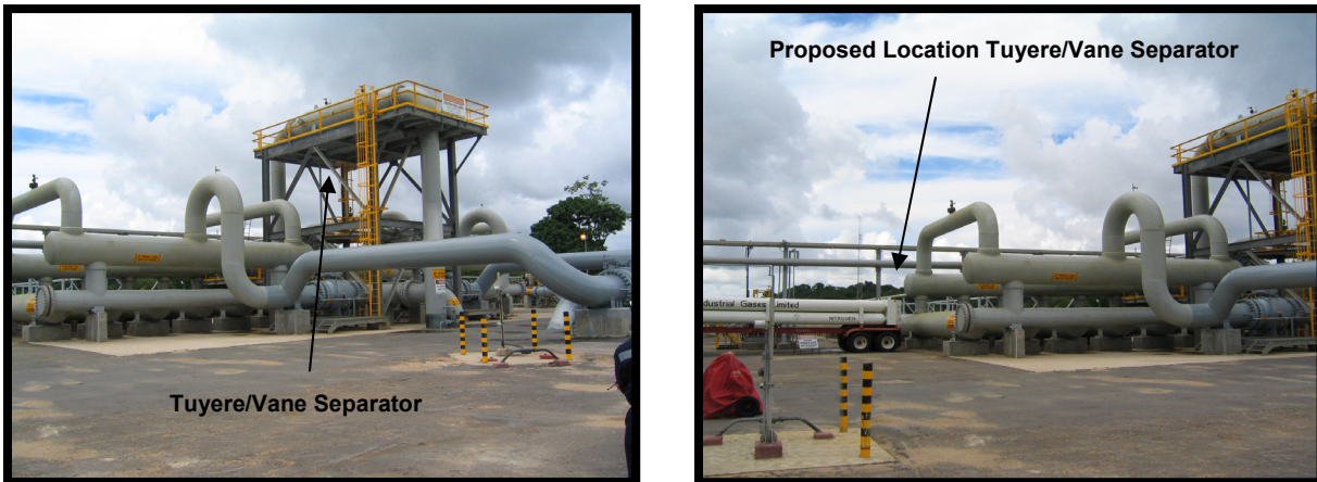
Figure 3.27: Location of Present and Proposed Tuyere Separators (Modification # 3)
