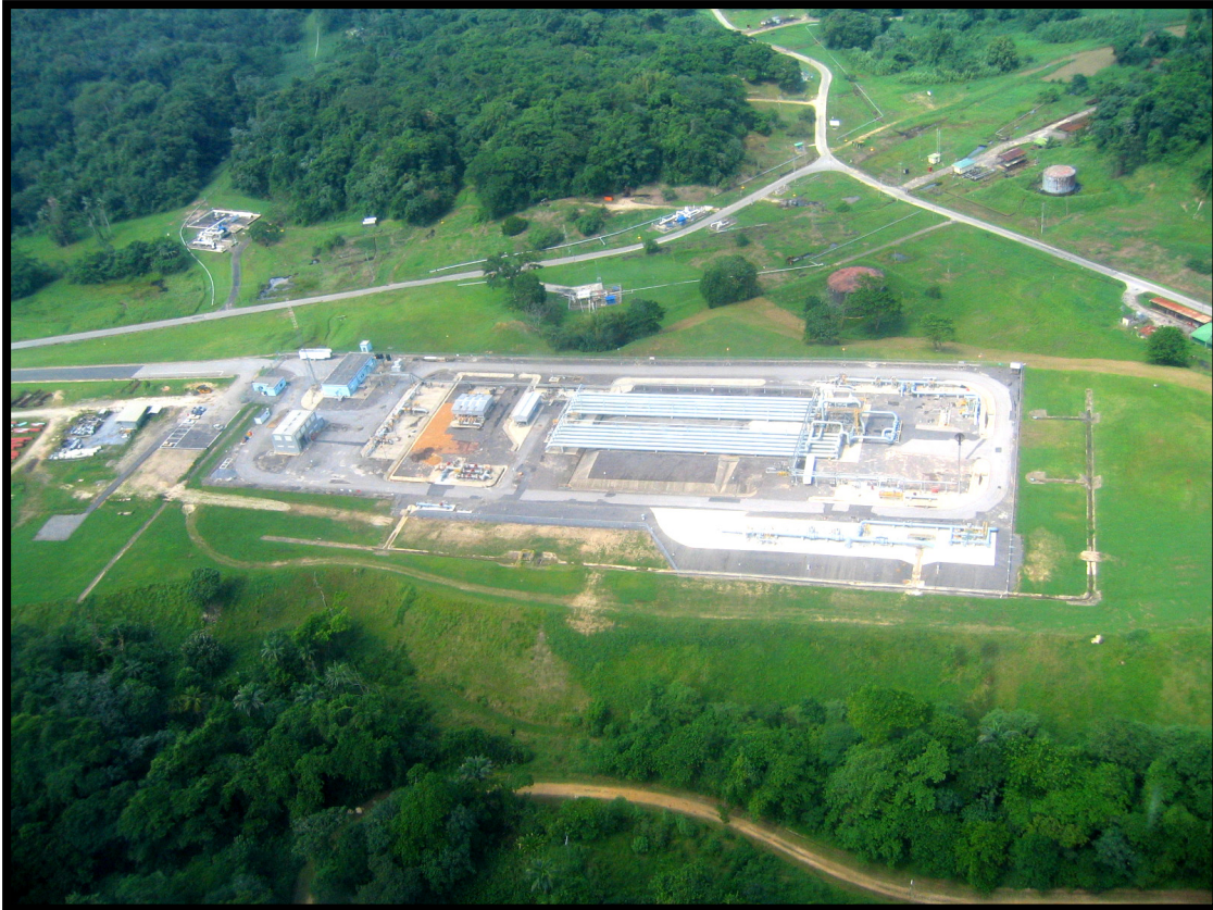
Figure 3.22: Aerial View of the Beachfield Gas Receiving Facility (from the southeast)
