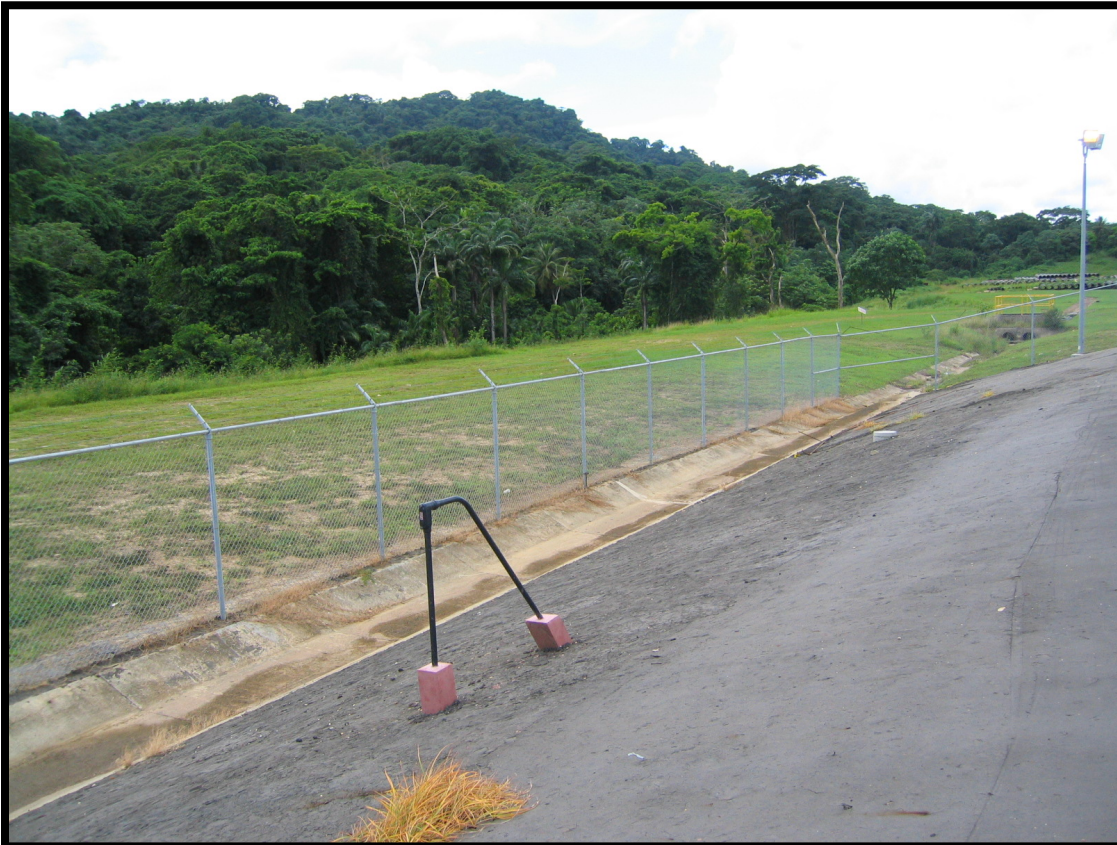
Figure 3.25: Area outside Beachfield Compound to be cleared for Pipeline.
