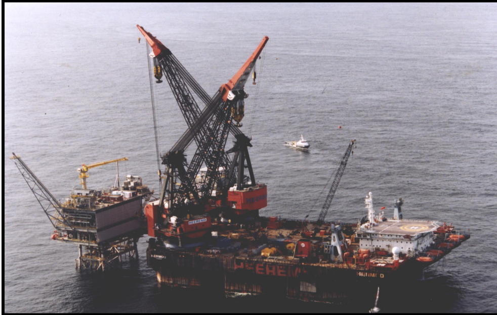
Figure 3.12: Installation of the Cassia “B” Hub in 2003
