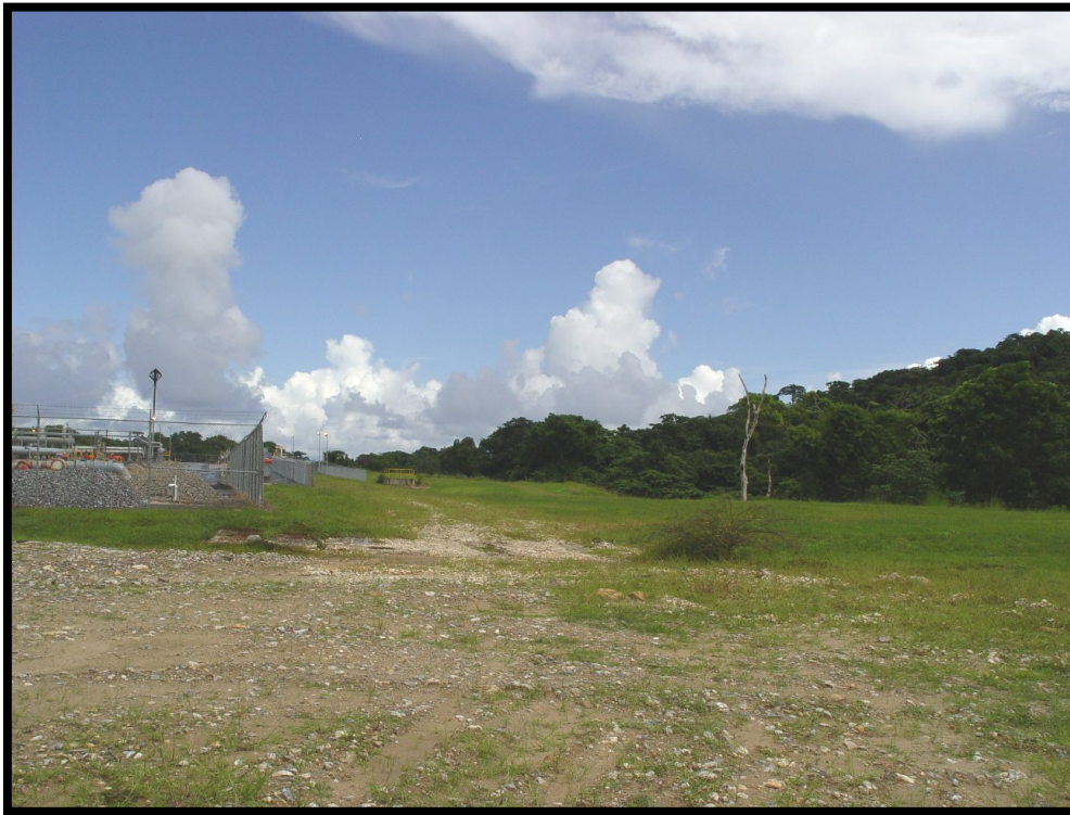
Figure 4.30: Beachfield Gas Receiving Facility
