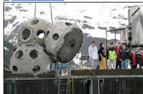
A group of school children watch as concrete balls weighing hundreds of pounds each, are lowered into the water at Smitty's Cove in Whittier, Alaska Wednesday May 10, 2006 to make Alaska's first artificial reef. The reef was in response to damage done when Alaska Marine Lines expanded its container facility at Whittier last year. (AP Photo/AI Grillo) (AI Grillo - AP)
