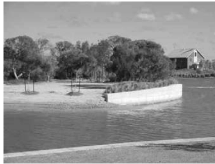
Figure 8. Example of beneficial mix of wall and sand intertidal habitat (Mariners Cove).
