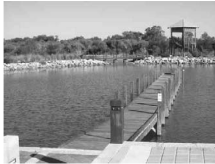
Figure 18. Photo of jetty at Mariners Cove that could be enhanced with Reef Balls.
