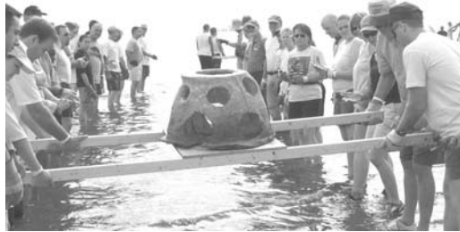
Figure 15. One method of transporting modules to shallow water reef sites. Photo courtesy of the Reef Ball Development Group.
