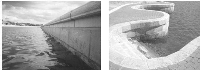
Figure 5. Photo of a typical straight canal wall, and another showing a variation is possible (Leeward and Eastport).
