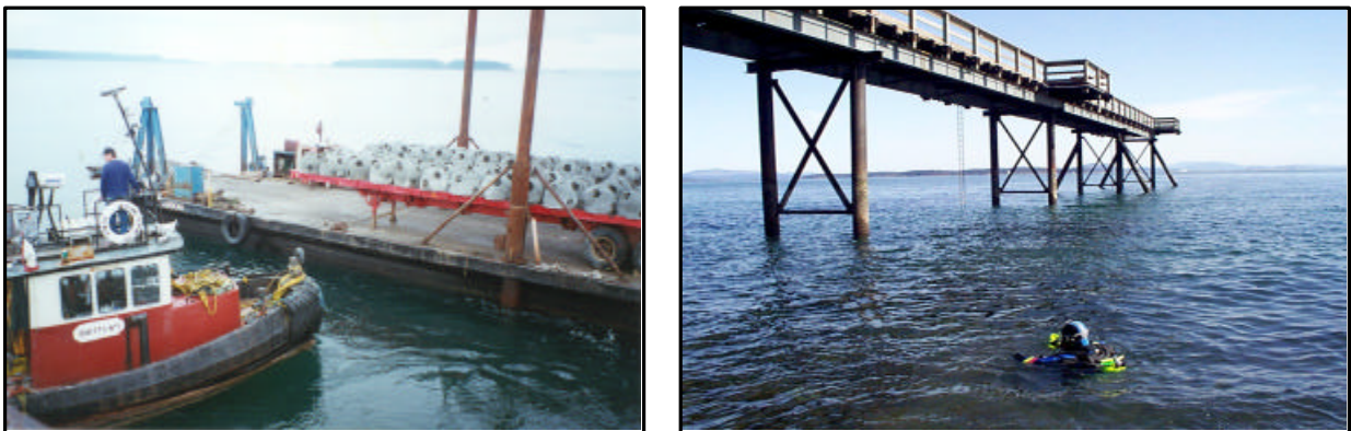
Figure 2. Reefball deployment off Sidney wharf, and diver showing landward entry point to Artificial Reef South (AS) just south of Sidney Pier.
