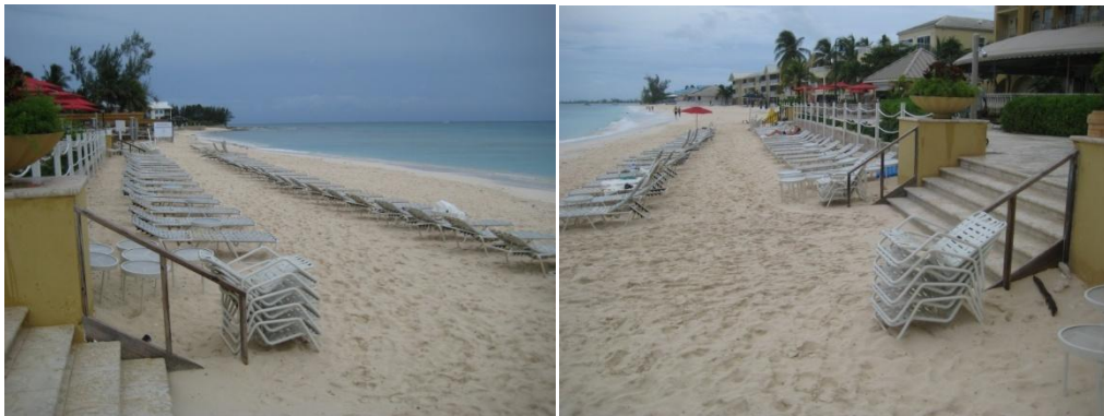
Figure C-8. View looking to the South and North at seawall in 06/08.
