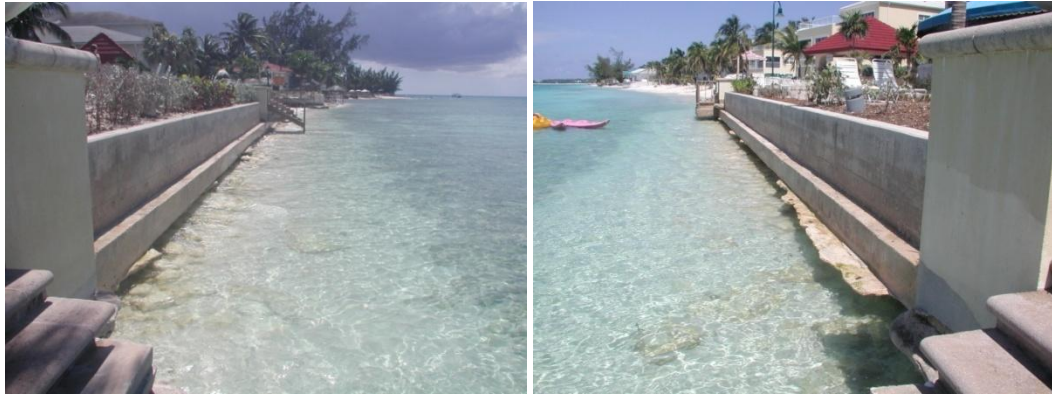
Figure C-4. View looking to the South and North at seawall in Oct. 2002
