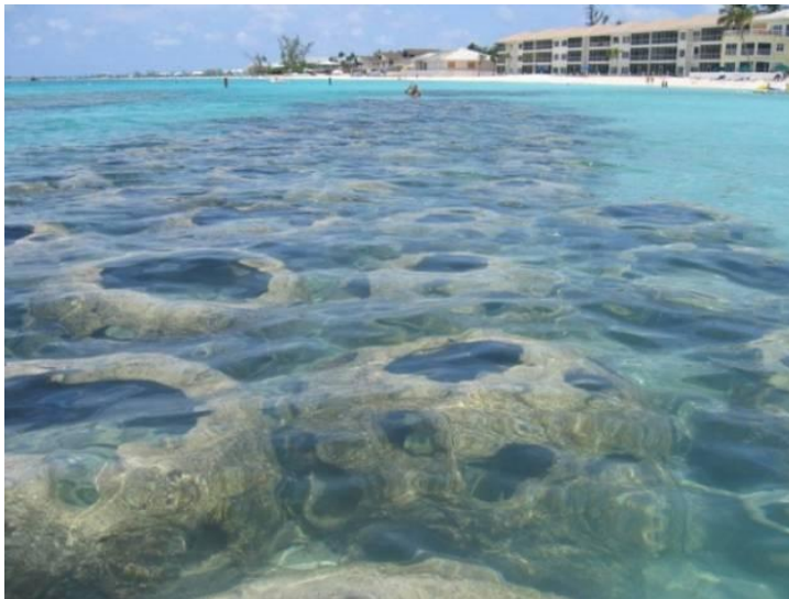
Figure 7. Reef Ball Breakwater after installation in Grand Cayman Island. (Photo courtesy of Lee Harris)
