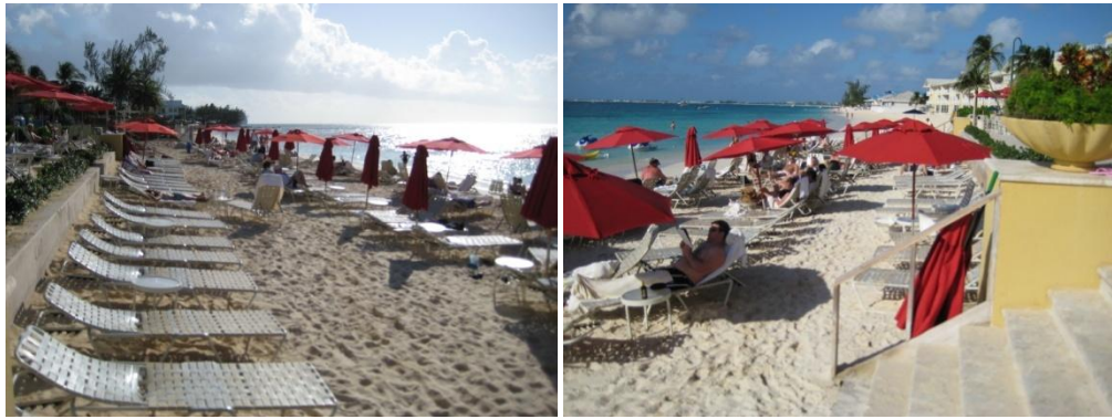
Figure C-7. View looking to the South and North at seawall in 01/08.
