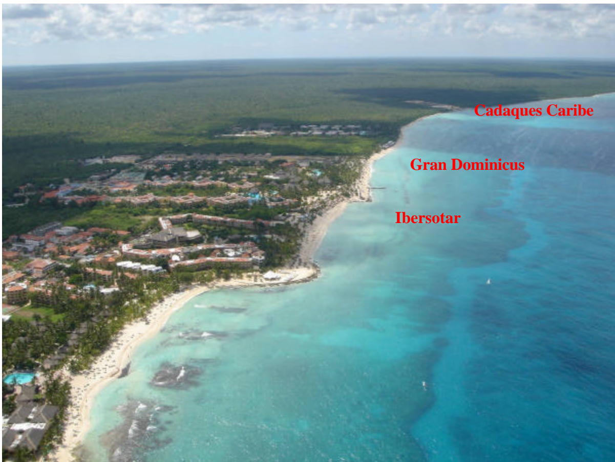
Figure 5. View East of Existing Submerged Artificial Reef Breakwaters
