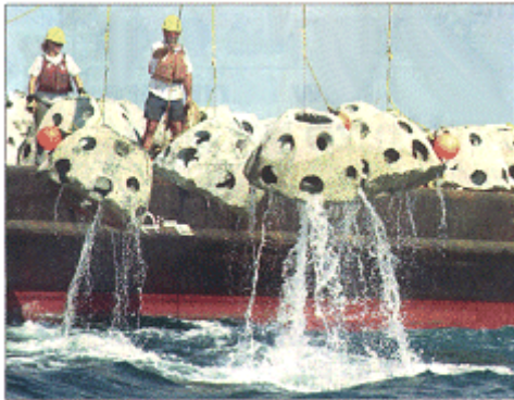
INTO THE SEA: Workers guide modules into the ocean off Dania Beach for a Nova Southeastern University Oceanographic Center project aimed at repairing a coral reef. Sun photo/Janis Stocker
