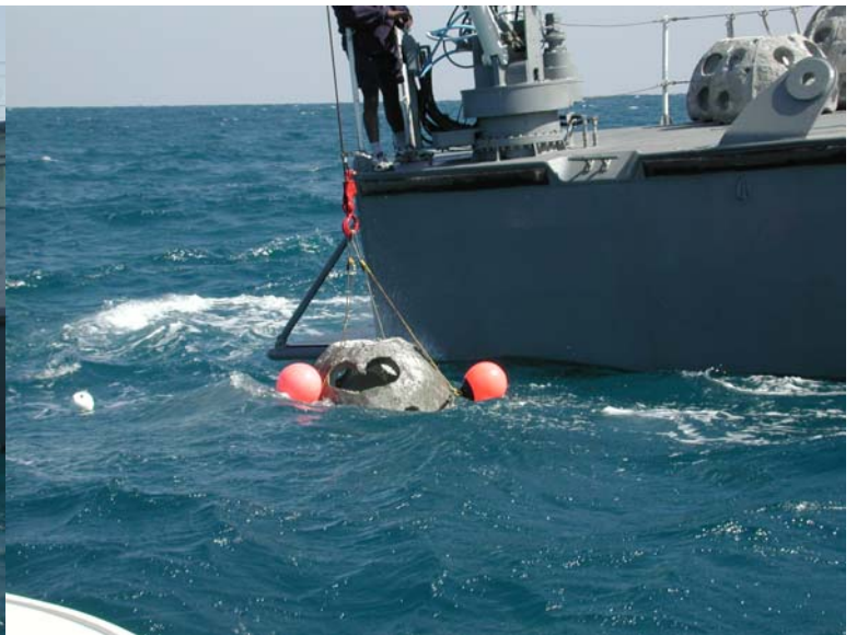
Lowering Reef Ball with buoy release mechanism. Note proximity to white target buoy.
