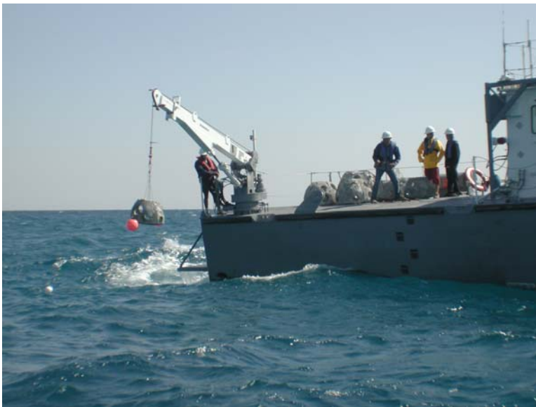
Reef Balls hoisted off deck by crane, lowered into position. Small white buoy serves as target.
