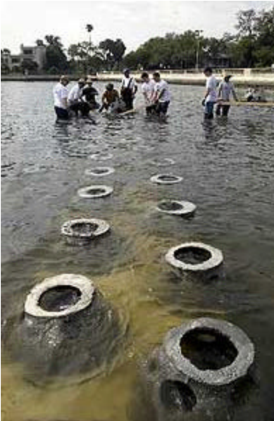
Photo by: JAY CONNER Volunteers install "oyster balls" near a sand spit near the southern end of Bayshore Blvd. Volunteers were there to install "oyster balls" to help protect the small beach from erosion.
