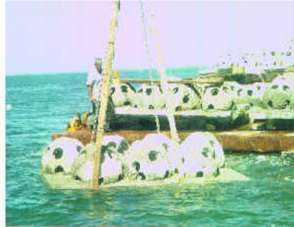
A load of reef balls made with FTR's RubberRock aggregate are deployed in Sarasota Bay. Reef balls create instant habitat allowing depleted fish populations to replenish themselves.
