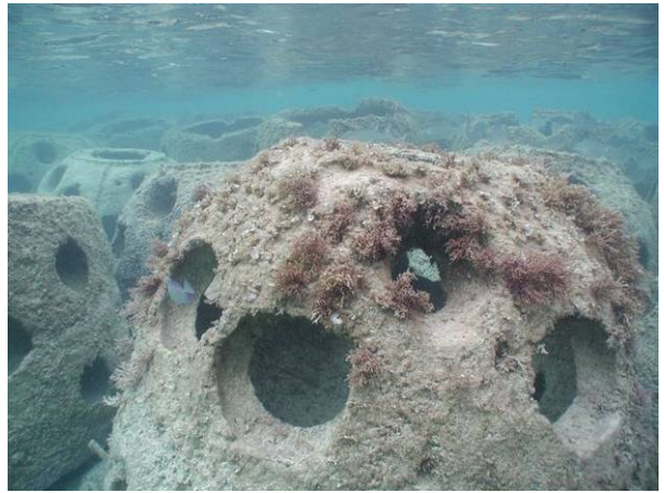
Figure 7. Five-Row Reef Ball Submerged Breakwater offshore of the Grand Cayman Marriott Beach Resort
