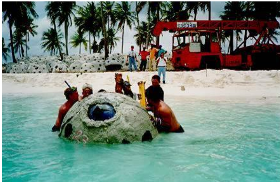
Figure 3. Deployment by Floating Reef Ball Units from Beach Fabricated units awaiting deployment can be seen in the background.
