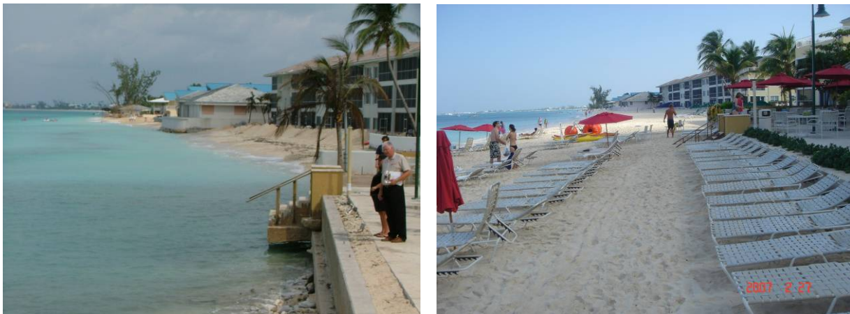
Figure 11. Marriott Beach before Reef Ball Breakwater Installation (on the left, Fall 2002) and after the Reef Ball Breakwater Installation (on the right, February 2007)
