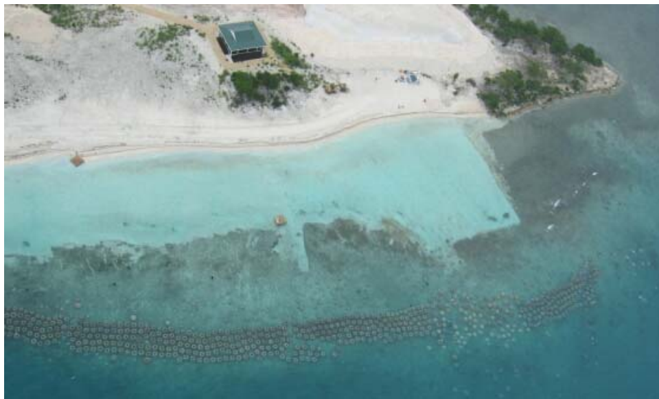
Figure 16. Aerial Photograph of 5-Row Reef Ball Breakwater in Antigua (The breakwater also incorporates snorkel trails, swimming and diving areas.)
