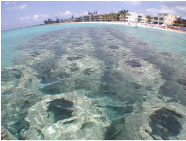
Figure 7. Five-Row Reef Ball Submerged Breakwater offshore of the Grand Cayman Marriott Beach Resort
