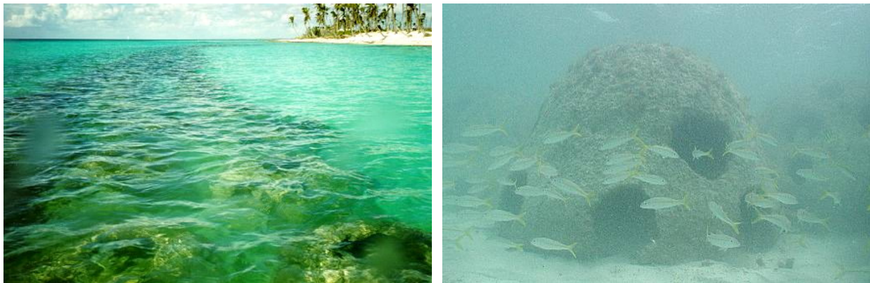
Figure 4. Gran Dominicus 3-Row Reef Ball Submerged Breakwater (Harris, 2003)
