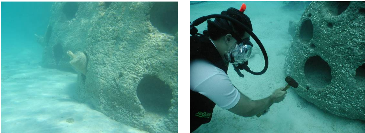
Figure 17. Pilings (left) and Rods (right) into Sea Bottom through Reef Ball Units
