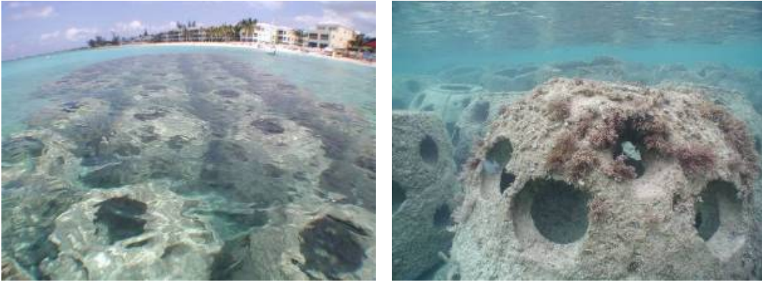
Figure 17. Above and Underwater Photographs of the Reef Ball Breakwater Submerged Breakwater offshore of the Grand Cayman Marriott Beach Resort
