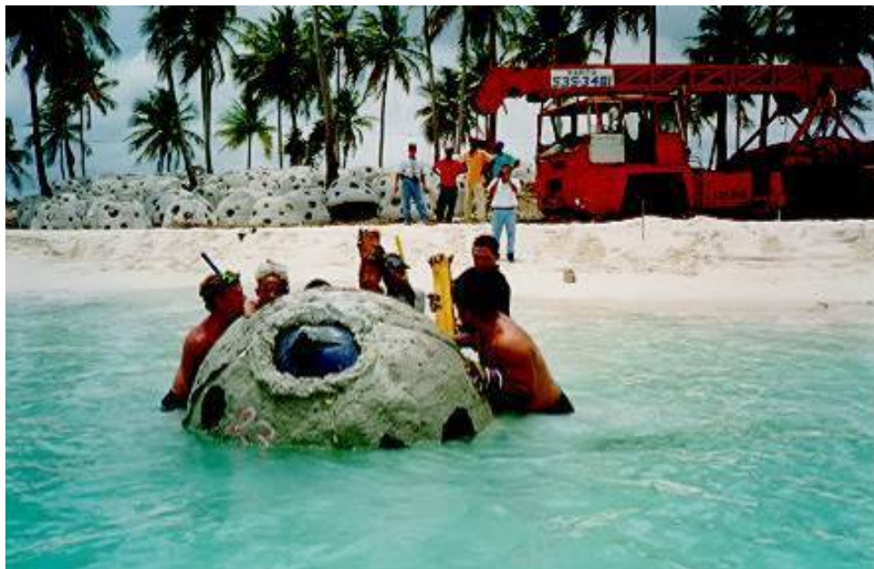
Figure 13. Deployment by Floating Reef Ball Units from Beach
