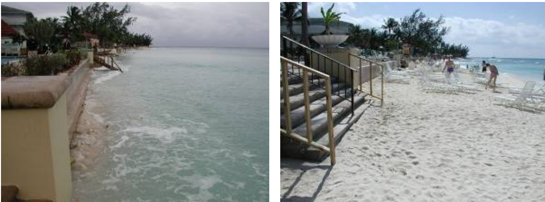
Figure 18. Marriott Beach Before and After Reef Ball Breakwater Installation Photo from Fall 2002 (L) and February 2003 (R) after the breakwater installation
