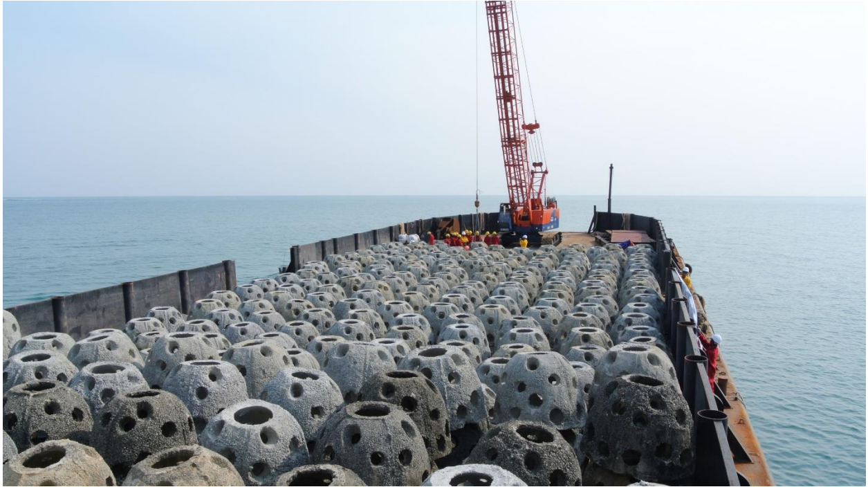
Figure 1. Reef Ball loaded on the vessel and ready for deployment
