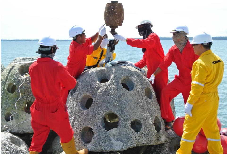
Figure 5. Installation of deployment sling and buoys on a reef ball
