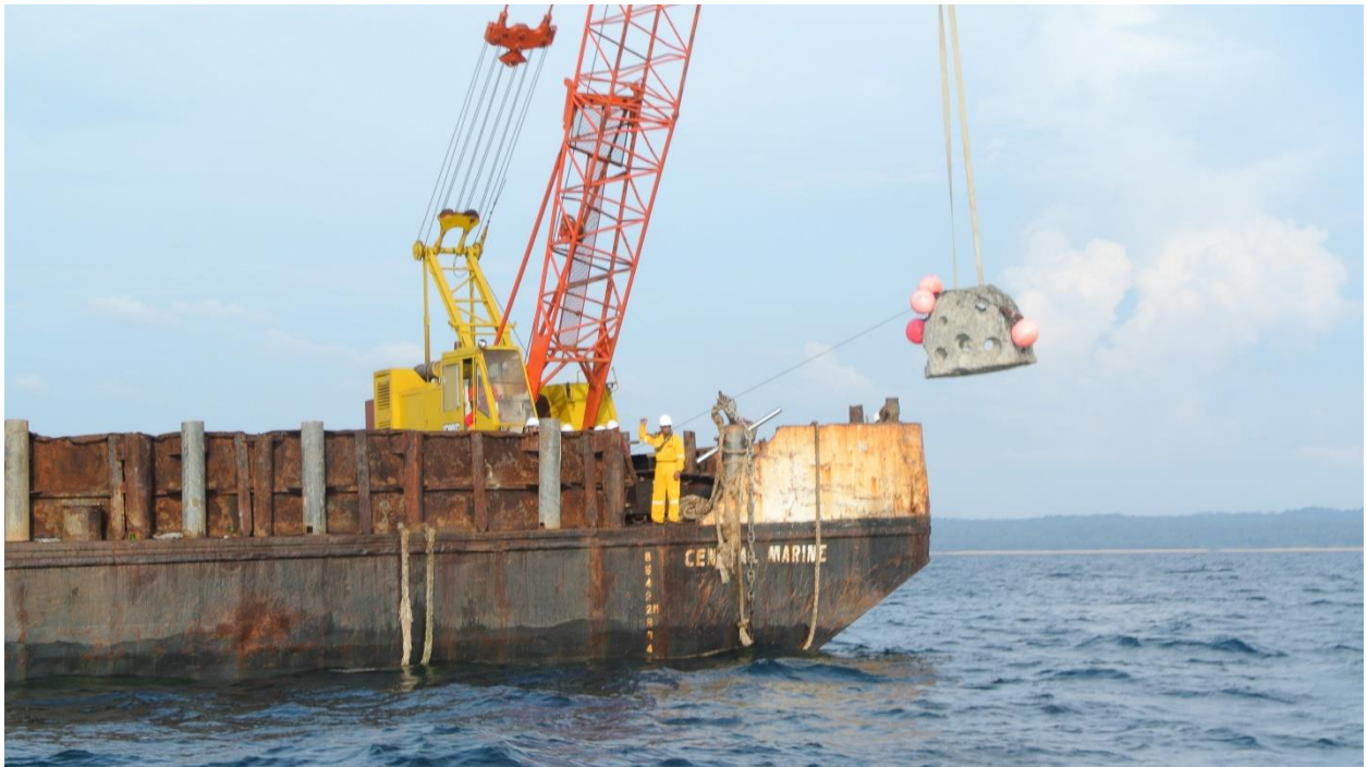
Figure 2. Reef ball being lowered down into the sea at the deployment site
