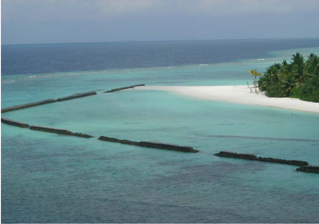
Plate 3-4: Breakwaters on north eastern side of the island and southern thundi joined with the breakwater on the southern end
