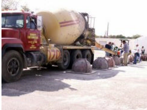
Pouring concrete in prepared molds
