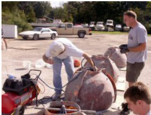
Pumping air into balls to create holes
