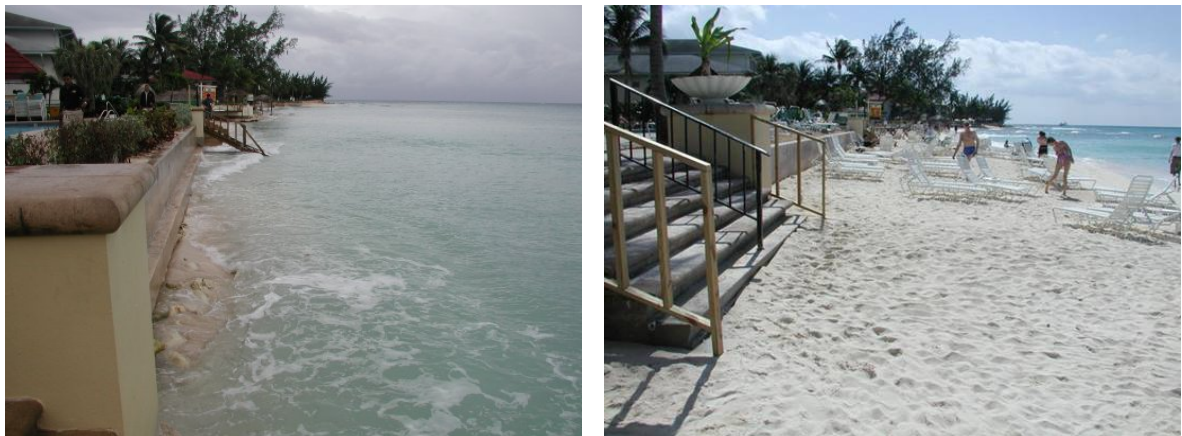
Figure 17. Grand Cayman Marriott before and after Reef Ball Breakwater Installation Fall 2002 on the left, February 2003 on the right.
