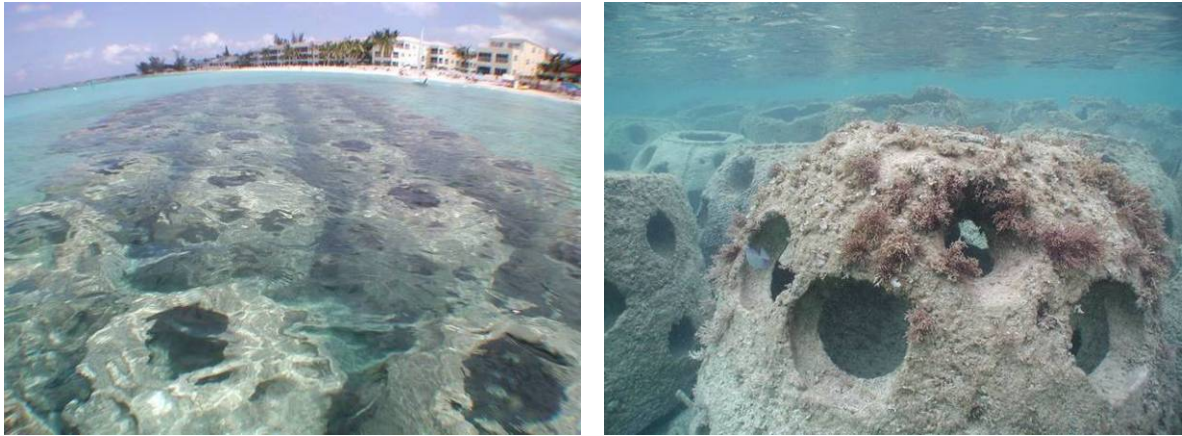
Figure 16. Grand Cayman Marriott Five-Row Reef Ball Submerged Breakwater
