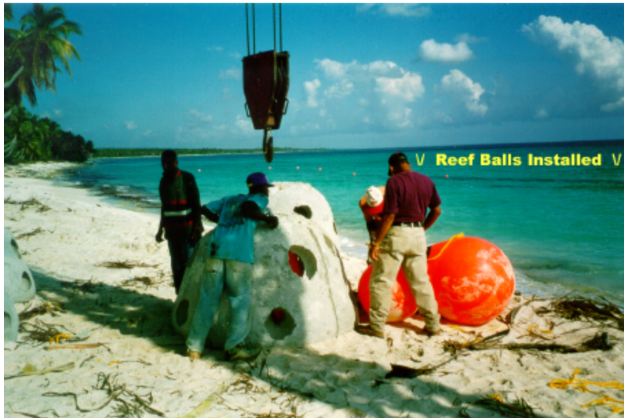
Ultra Reef Balls being deployed at Gran Dominicas Hotel in the Dominican Republic, note the appearance of the Reef Ball submerged breakwater as only a dark line in the water. This would be the same look generated at the Mayan Palace.
