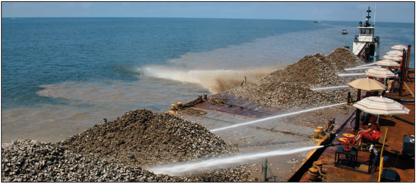
DMR Shellfish Bureau staff use high-pressure hoses to spread oyster shells onto reefs near Pass Christian.
