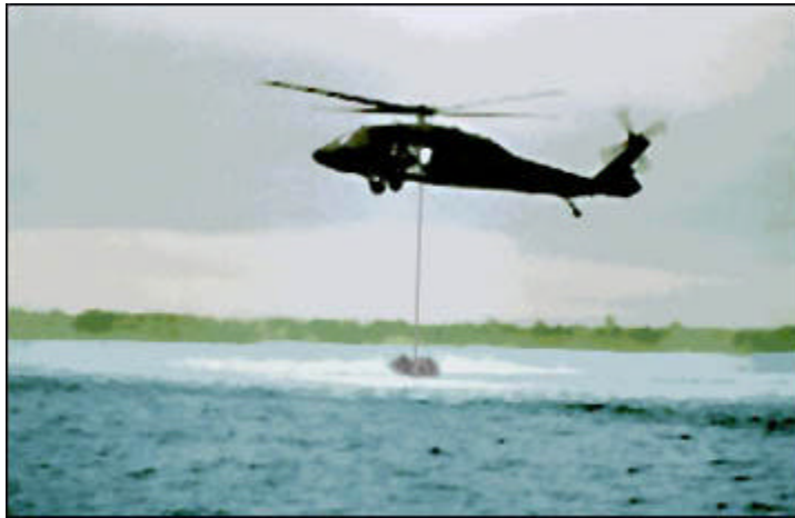
Placing Reef Balls along DEC Panels
