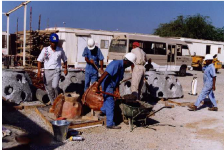
Fabrication in full swing
