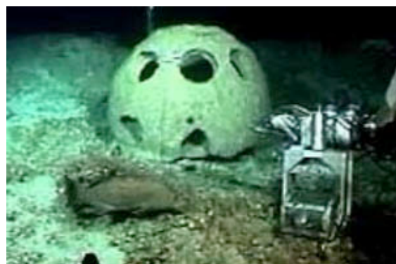
Fig. 7. Artificial reef structure for implementation of juvenile corals
