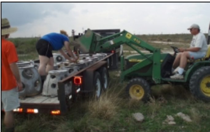
Eddie Seidensticker (NRCS) drives the front-end loader used to relocate the reef balls to the shoreline for deployment.
